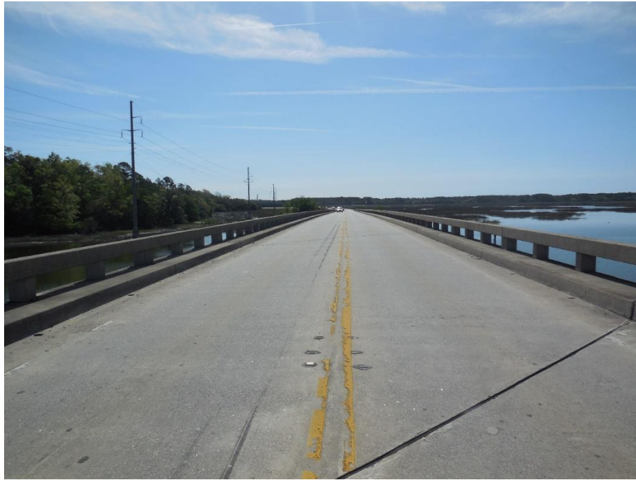
SR 204 Spur EB MP 4.82, Before
